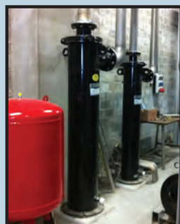
Cleaning chilled water, Axima Belgium
